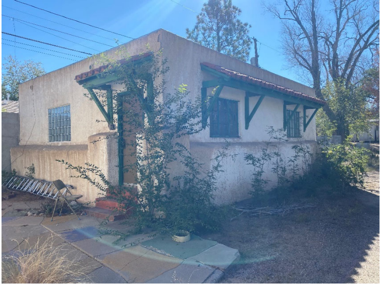
Figure 5: Rental unit # 2, door and awning details.
