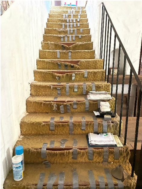
Top left: caving ceiling in main house; bottom right: deteriorated stairs in main house; bottom left: non-compliant stairs leading to 2 nd floor deck.
