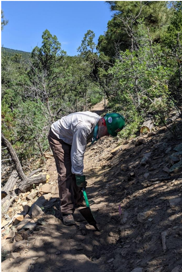
Re-benching down towards the junction
