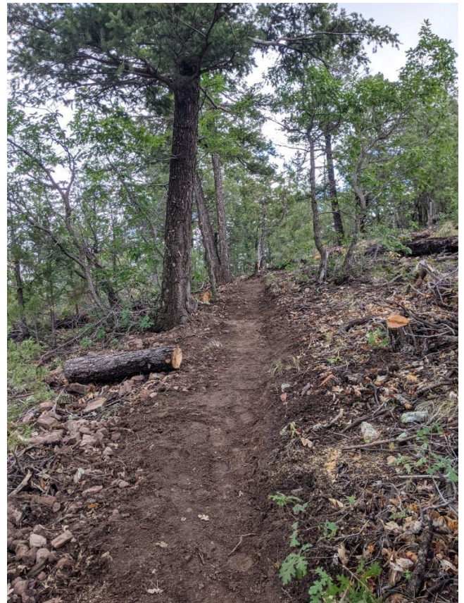
Part of the new connecting section on Vista
