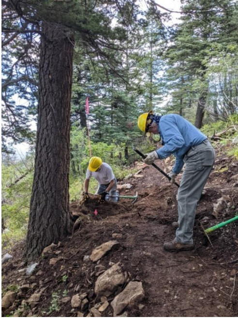
Shoring up the tread
