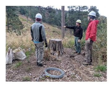
Deciding what to move with the griphoist. You can see the wire rope in the foreground, which will be threaded through the griphoist. The bags hold other accessories. It takes time and a good deal of thought to prep the object being moved, before setting up the griphoist.
