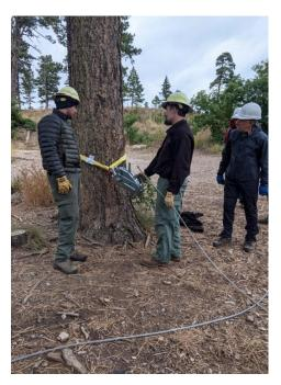
The griphoist is attached to the anchor and the wire rope gets threaded through it.
