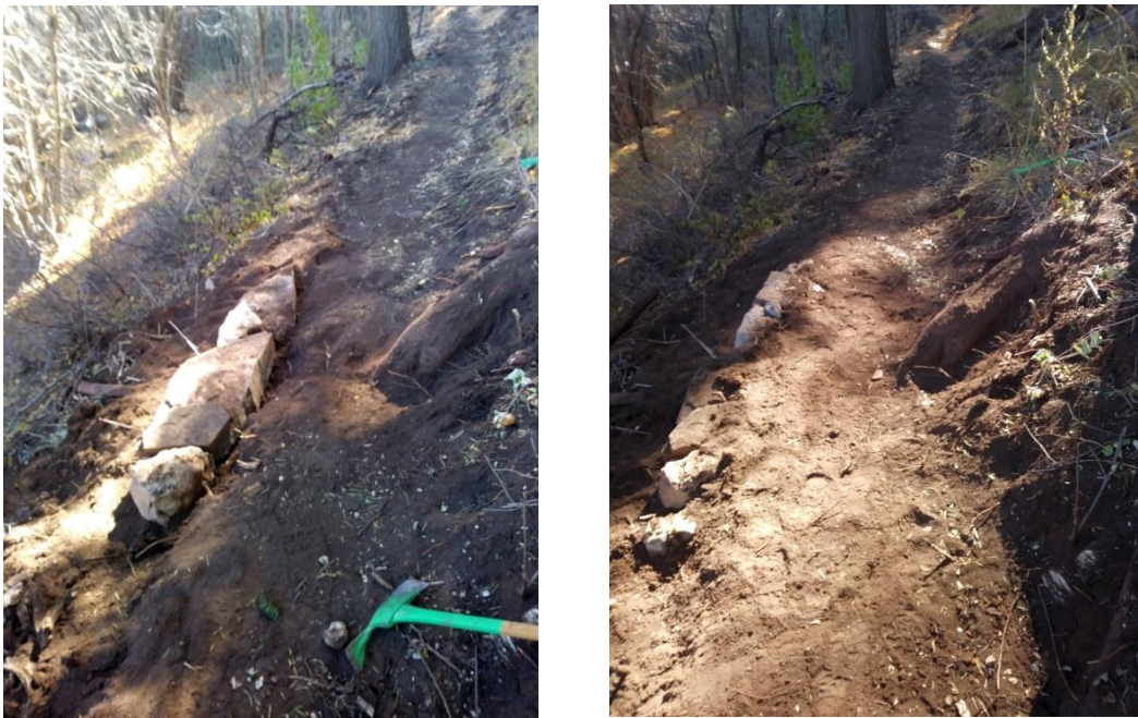
During and after, looking south
