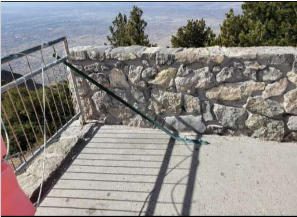
The right end of the railing was easy to secure, once the fencepost was cut, bent, and drilled.
