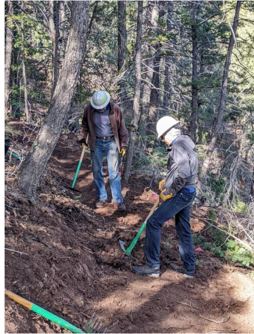
Some work on a previous section
