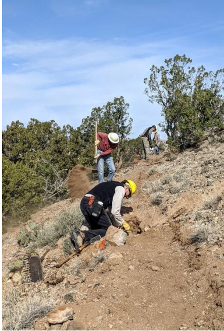
Sim finds a section that could use some rock cribbing. (Jeff and Byron in background, Byron dispersing dirt)
