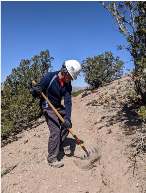
At location 2, Luis works to widen the tread
