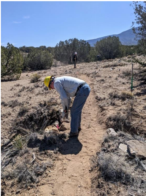
Eric shores up the trail where it crosses a wash
