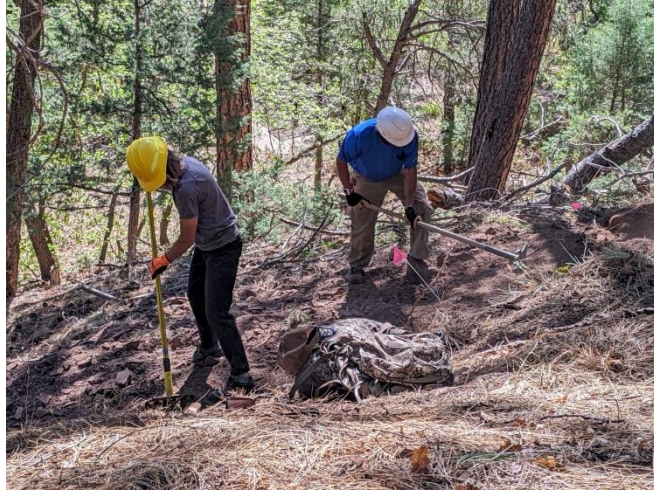
Pat and Jeff have cleared the duff. Now they're benching in new tread.
