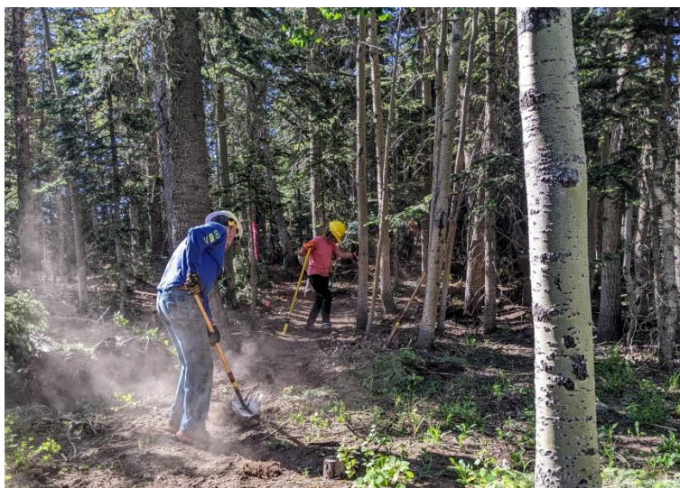
Jim and Pat near the beginning/north end of the new extension
