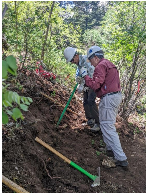
Ed and David ponder how building the backslope can sometimes be the toughest part!
