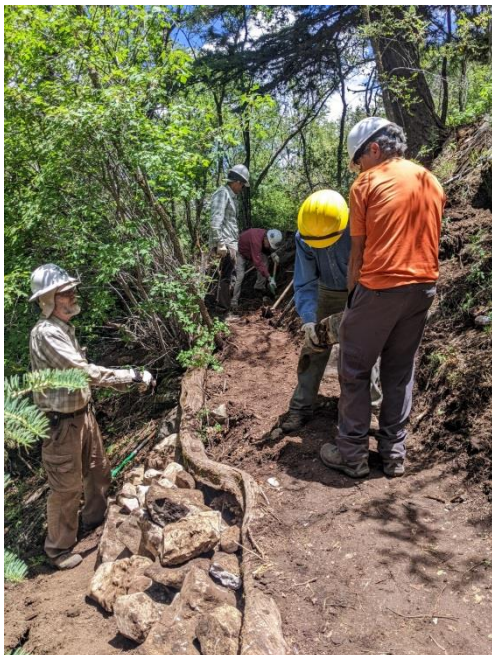
Eric and Luis share the load. Bruce takes his turn below the tread. David and Ed continue knocking back the backslope. (The crib wall remains a work in progress. Next session!)
