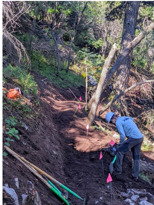
The Maddens work on the backslope while David widens a section of tread
