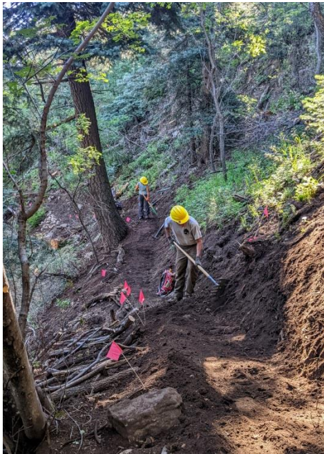
The Maddens work on the backslope while David widens a section of tread
