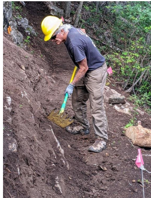
Mike works on the backslope
