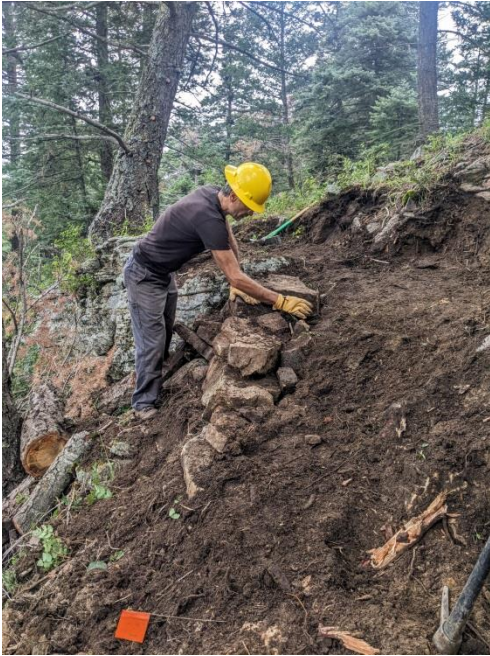
Roland and Mark (not in photo) build a short retaining wall
