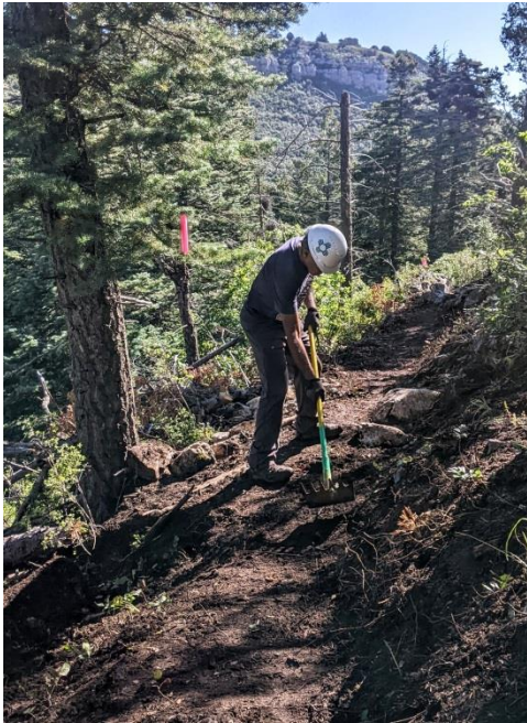
Luis builds a drainage feature
