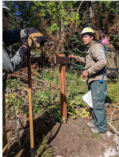
Joseph and the relocated Switchback Trail sign. What arrow...?
