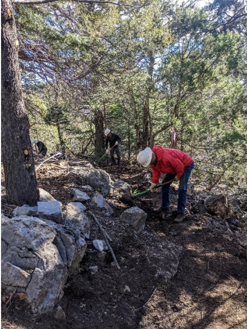
Bruce removes a rock from the backslope (Tony, Scott)
