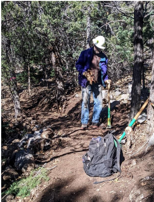
Jim pulls an old root from the backslope (and many large rocks)
