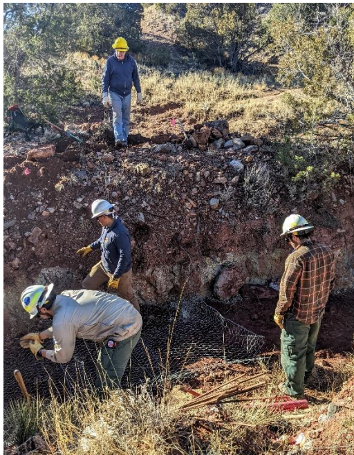
Russell, Jeff C and Joseph start assembling a cage for the first gabion. Eric observes from the perch which he later transforms.
