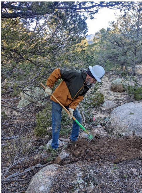
Bruce gets started near the east (uphill) end of the reroute
