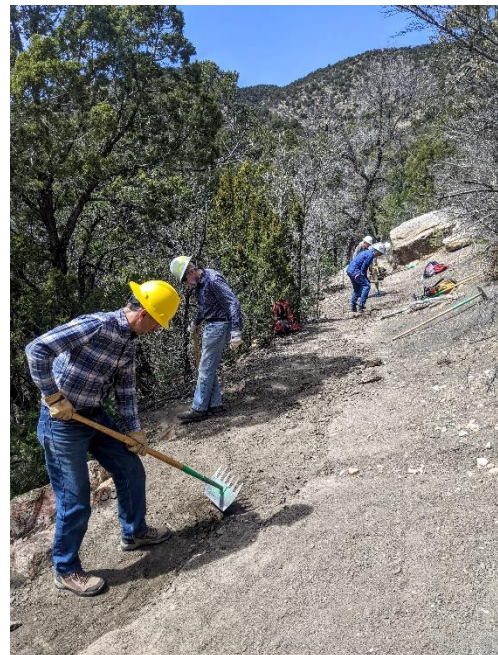
On the hike out the crew spends time rebenching an out-sloped section near the trailhead.
