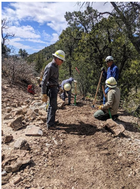
Sim, Byron and Luis have moved rocks onto the old tread (left) to create the reroute (right). Joseph consults.
