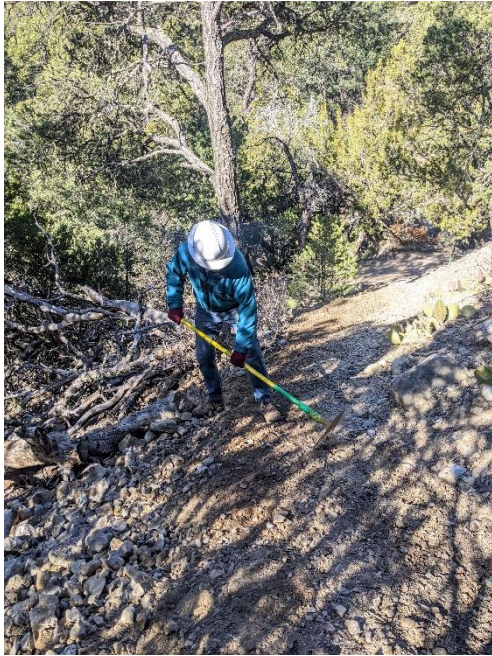
Bill puts some finishing touches on a section near the junction
