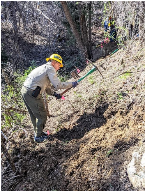
John and Bill get their first taste of benching on steeper sideslope (Scott in background)
