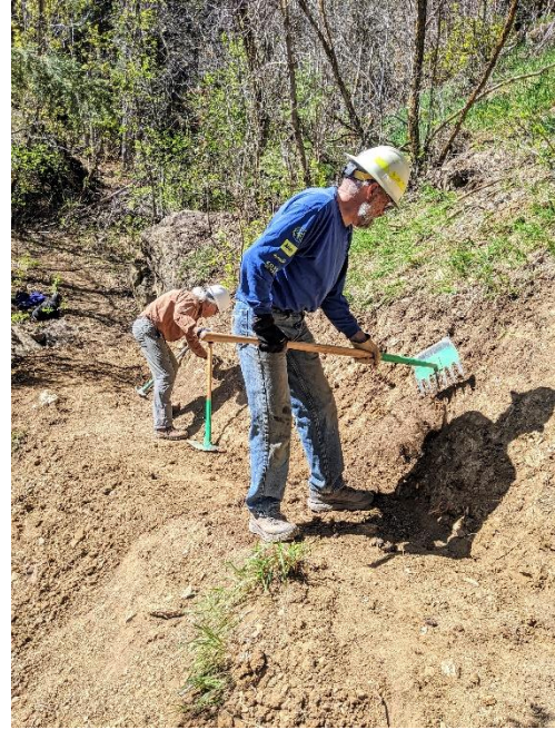
Finishing the backslope Jim, Bill
