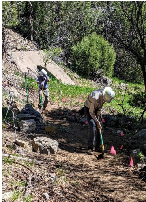
Sim and Bill approach the culvert. This is the small one!
