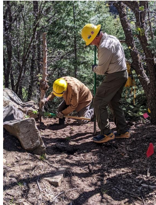
The rock can stay. Dan starts digging.
