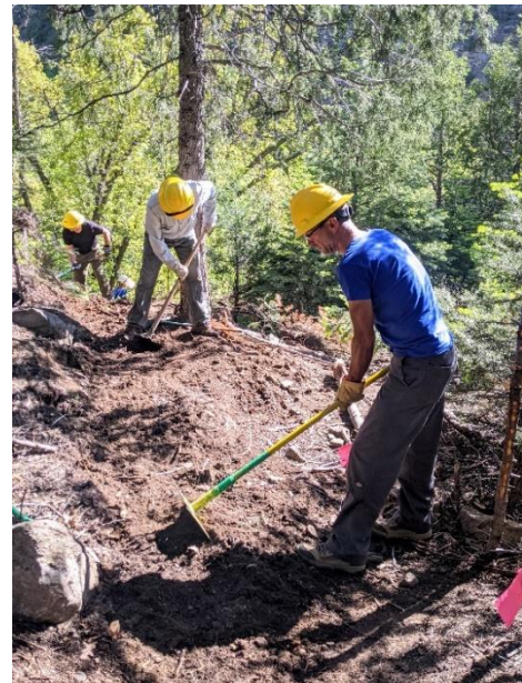
Roland, Eric and John work on one of Kerry's realignments
