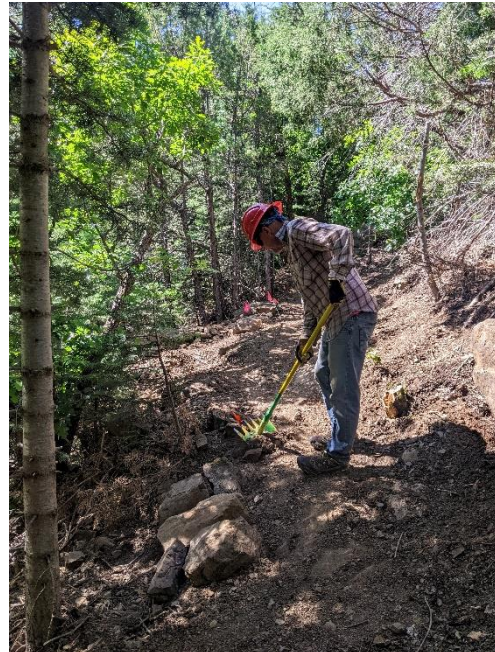
Claudia builds tread to the south. Tayo adds drainage farther north.
