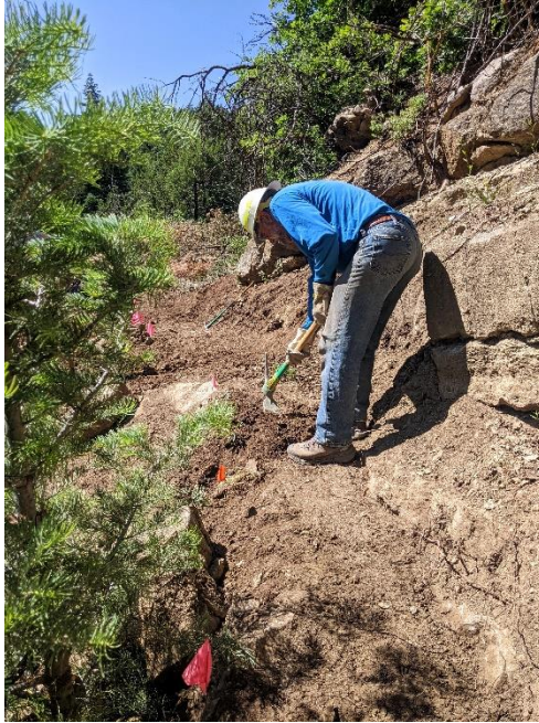
Jim builds new tread in a tight spot close to a bedrock wall
