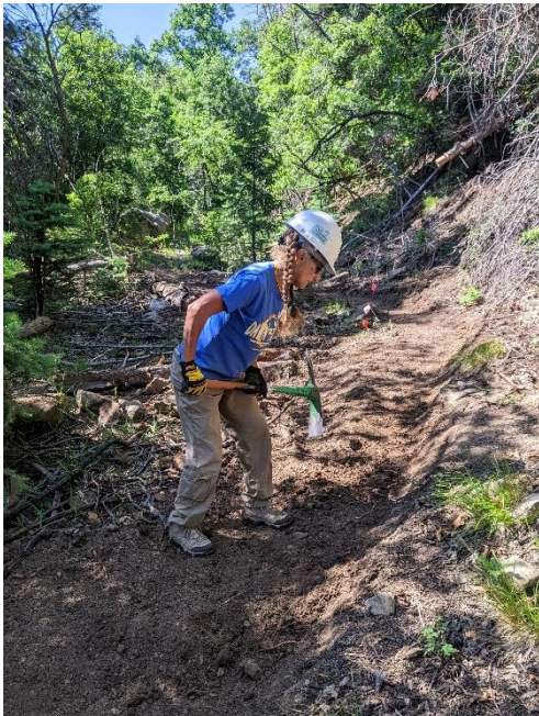
Claudia builds tread to the south. Tayo adds drainage farther north.
