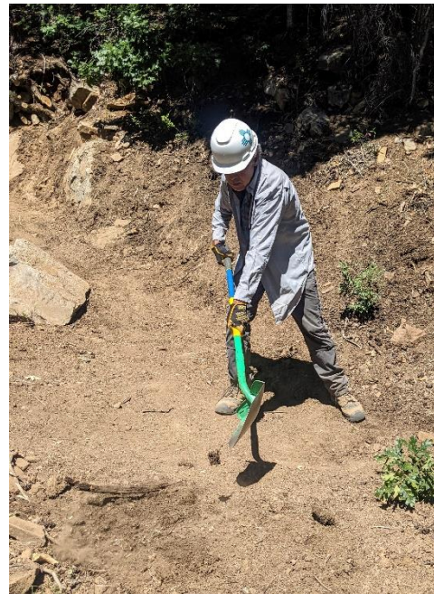
Luis works on drainage, happy for a shovel
