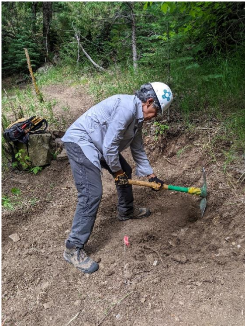
Luis works just west of the drainage
