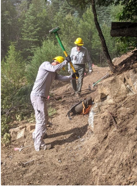
Swing it Joe! Sometimes backslope work = sledge work
