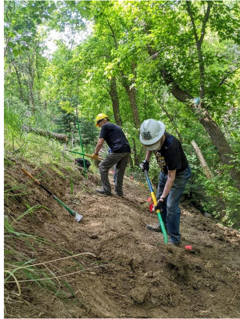
Dan and Bruce (and Jim) move dirt. So. Much. Dirt.
