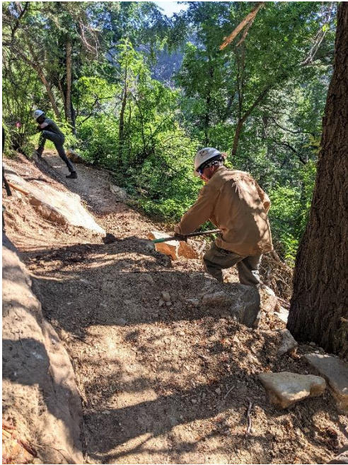
Crib work. Mugzy prepares the base below the outer edge of the tread. Needed: large rocks.
