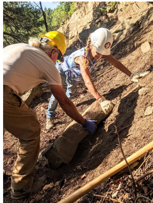
Mike and Claudia work on the backslope
