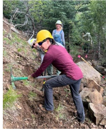
Jenny Blackmore and Kerry Wood using pick mattocks to build a segment of the Challenge Trail extension
