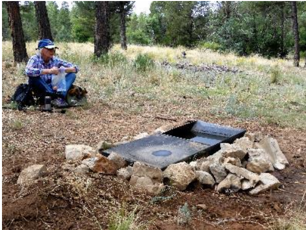
Joelle Hertel having lunch at the David Canyon East wildlife drinker. The float valve is in the steel box on the left, wildlife drink water from the open right side of the drinker.
