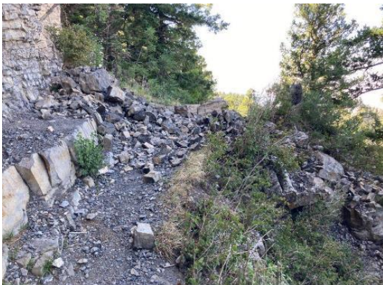
Crest Spur Trail rock fall looking South
