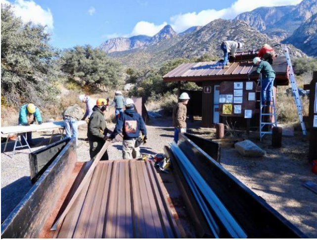
Installing a steel roof on the La Cueva Picnic Area restroom
