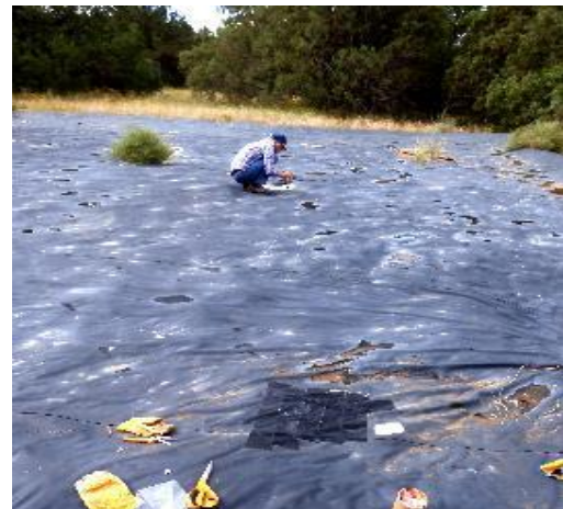
Joelle patching the David Canyon East rain collector fabric with black tape. Rain falls on the fabric and flows down to one corner where the water enters a pipe and goes to a storage tank.
