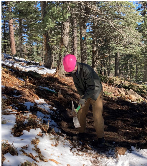
Roland Benching Trail
