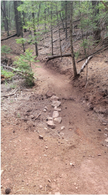
When dry extensive erosion of the trail as well as debris noted on outflow
