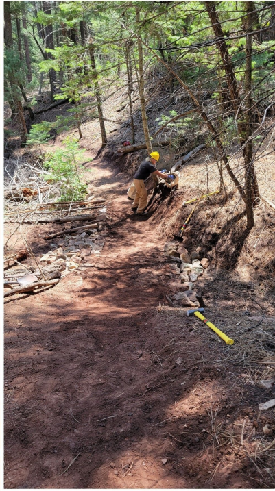
The top layer is soil brought in from either side of the trail
