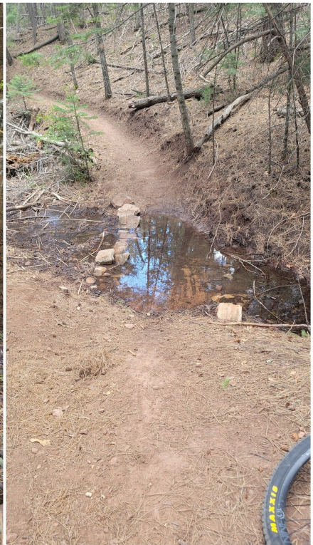
Resulting in a muddy drainage crossing leading to erosion
