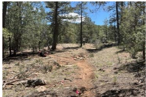
New trail to the left and old trail obliterated to the right with a check dam
