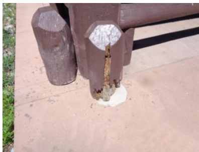
Post repair, before...
