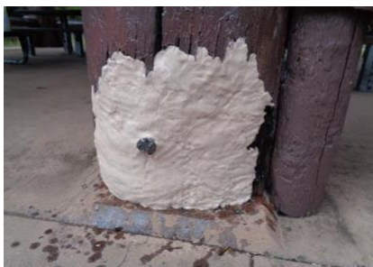
Max Putty has been applied to the decayed void on this column; putty is smoothed with fingers or palm and is painted brown after it has cured
