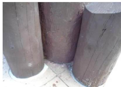
The lower 12-inches of the column between the two short posts has been treated with System Three products to fill the decayed void and painted brown
