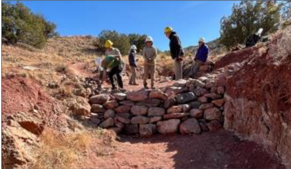
The Thursday trail construction & reroute crew hard at work: Rock work on the entrance to the Piedra Lisa trail
