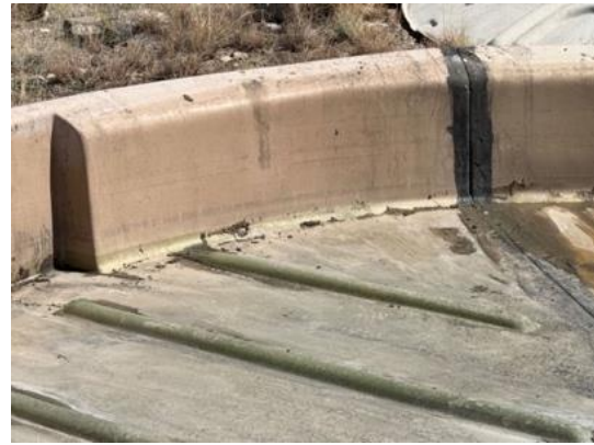
Open Basin Joint Sealed with Silicon
