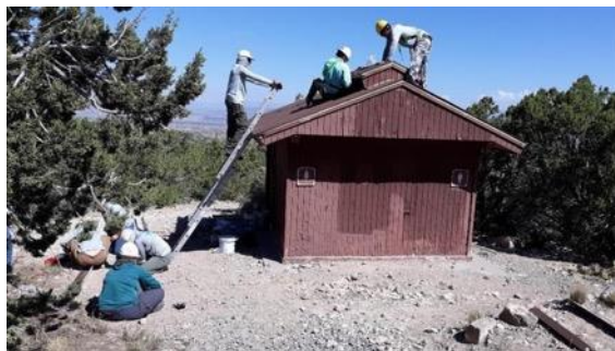
A New Metal Roof, Tunnel Spring Restroom
