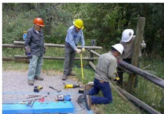
Attaching Poles to a New Post
