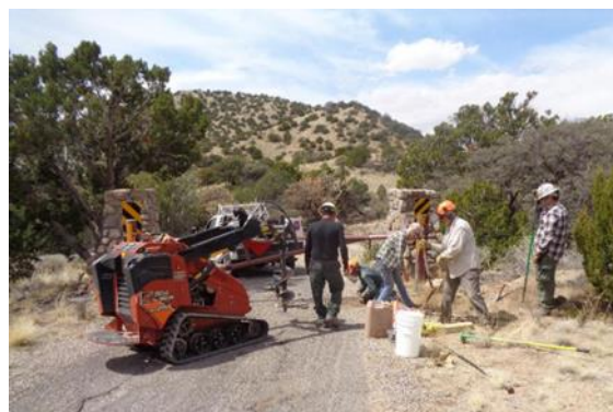
Installing New Steel Bollards at Juan Tabo PA Exit
