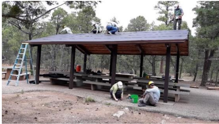
Installing a New Steel Roof, Yucca Shelter
