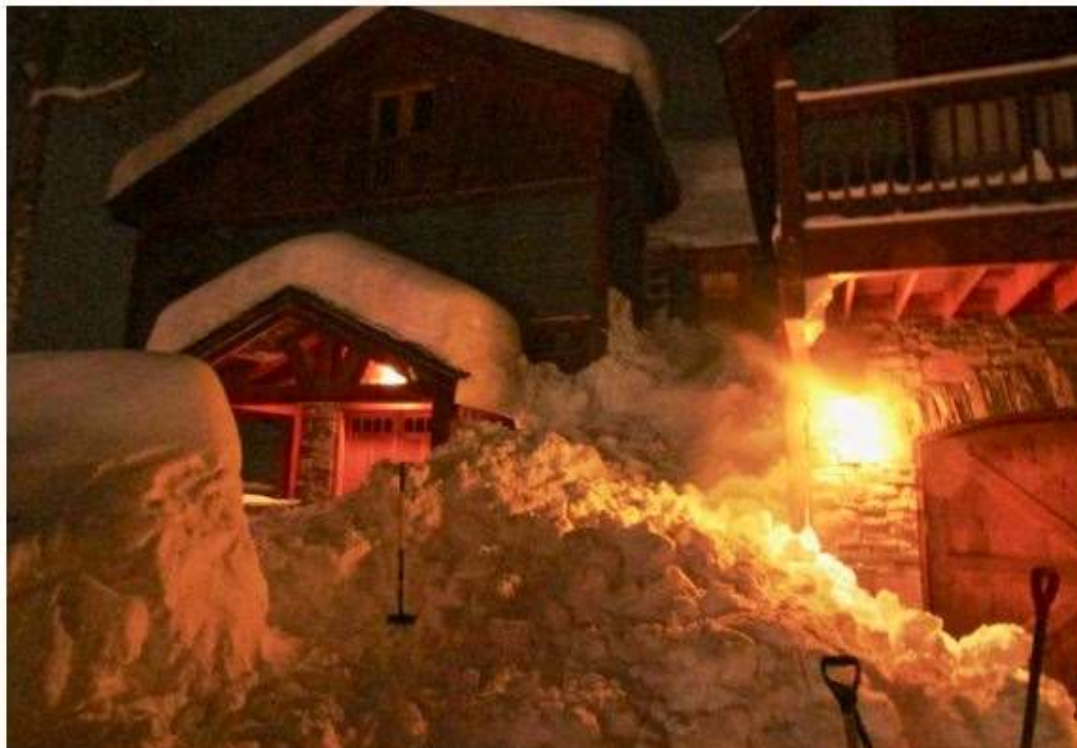
Figure 1: This roof avalanche caught and buried a person on March 8, 2019, in Mount Crested Butte. The avalanche came off the roof in the upper right, and the person was buried near the shovel on the left. ( see full sized image )
