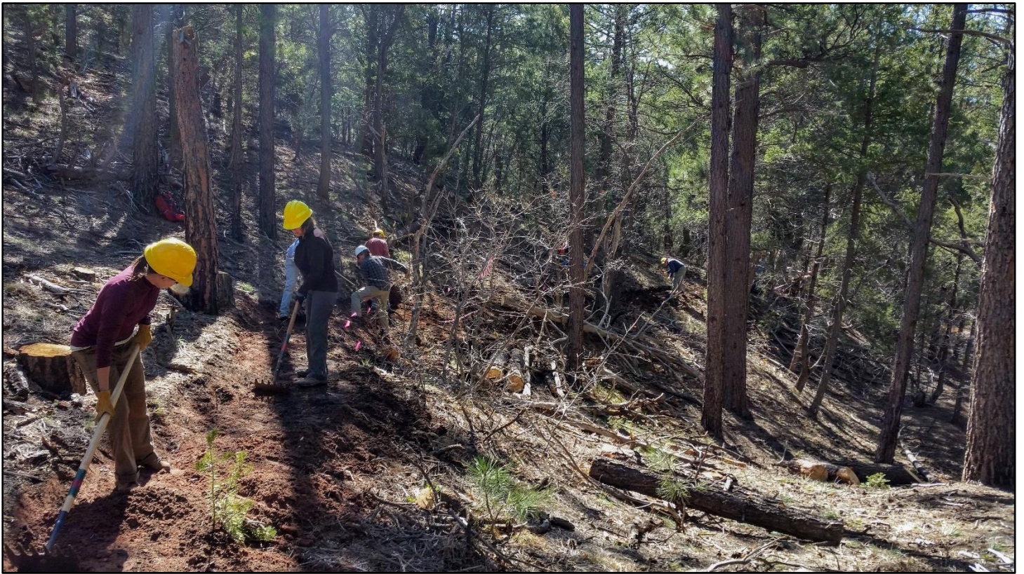
Coming out of open ponderosa forest, the crew worked into denser growth lower on the reroute.
