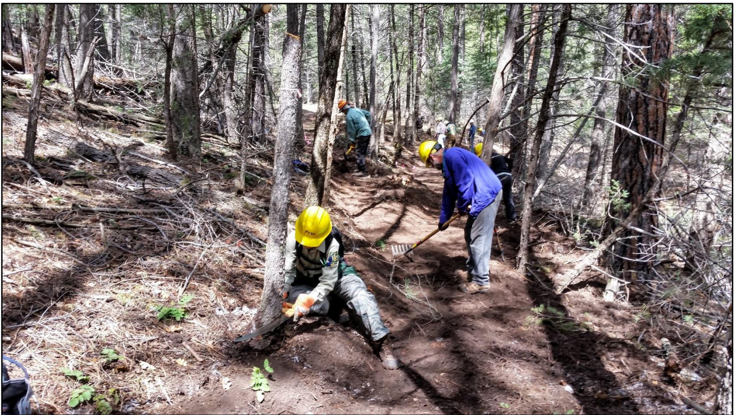
The final line missed a few stumps which luckily could just be low-stumped.
