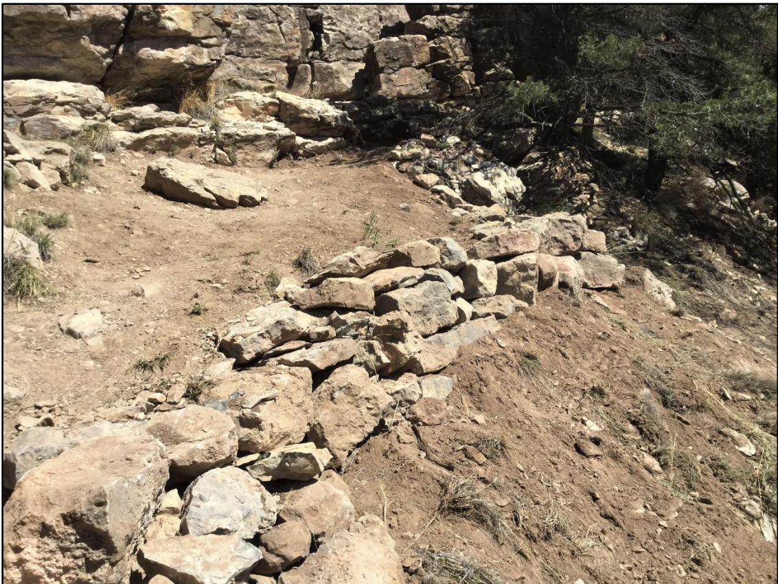
A crib and fill project improved this belay platform.
