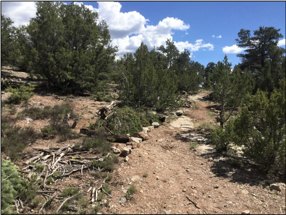
New tread and thinning slash serve to define the upper trail and guide trail users.
