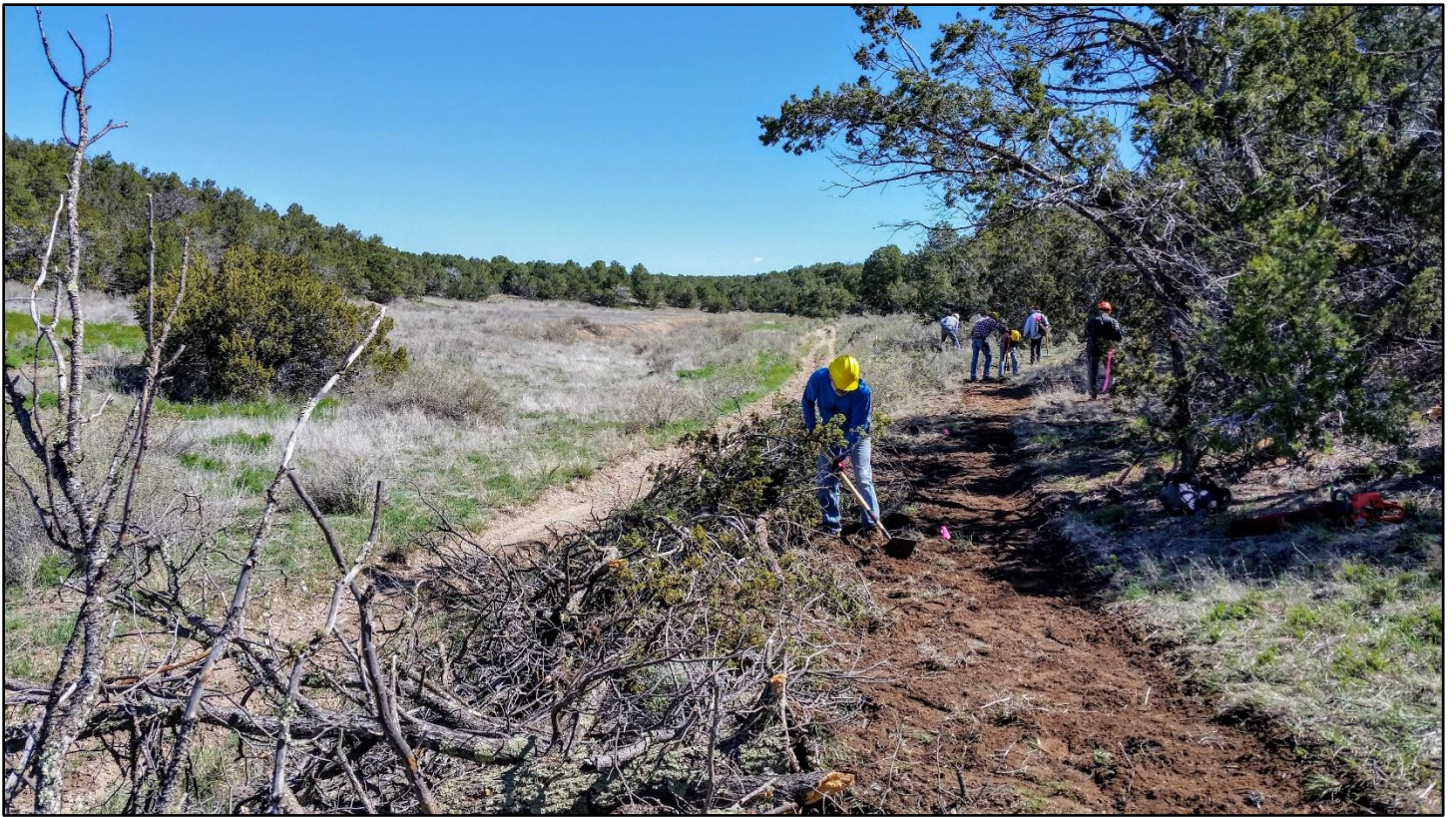
The old line was straight down the canyon and deeply rutted. This new line is a real trail.
