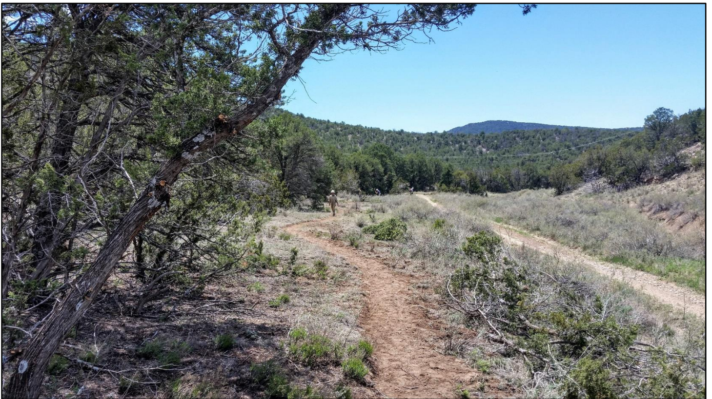
The boss picked an undulating line for drainage and to bring the trail up near the tree line.
