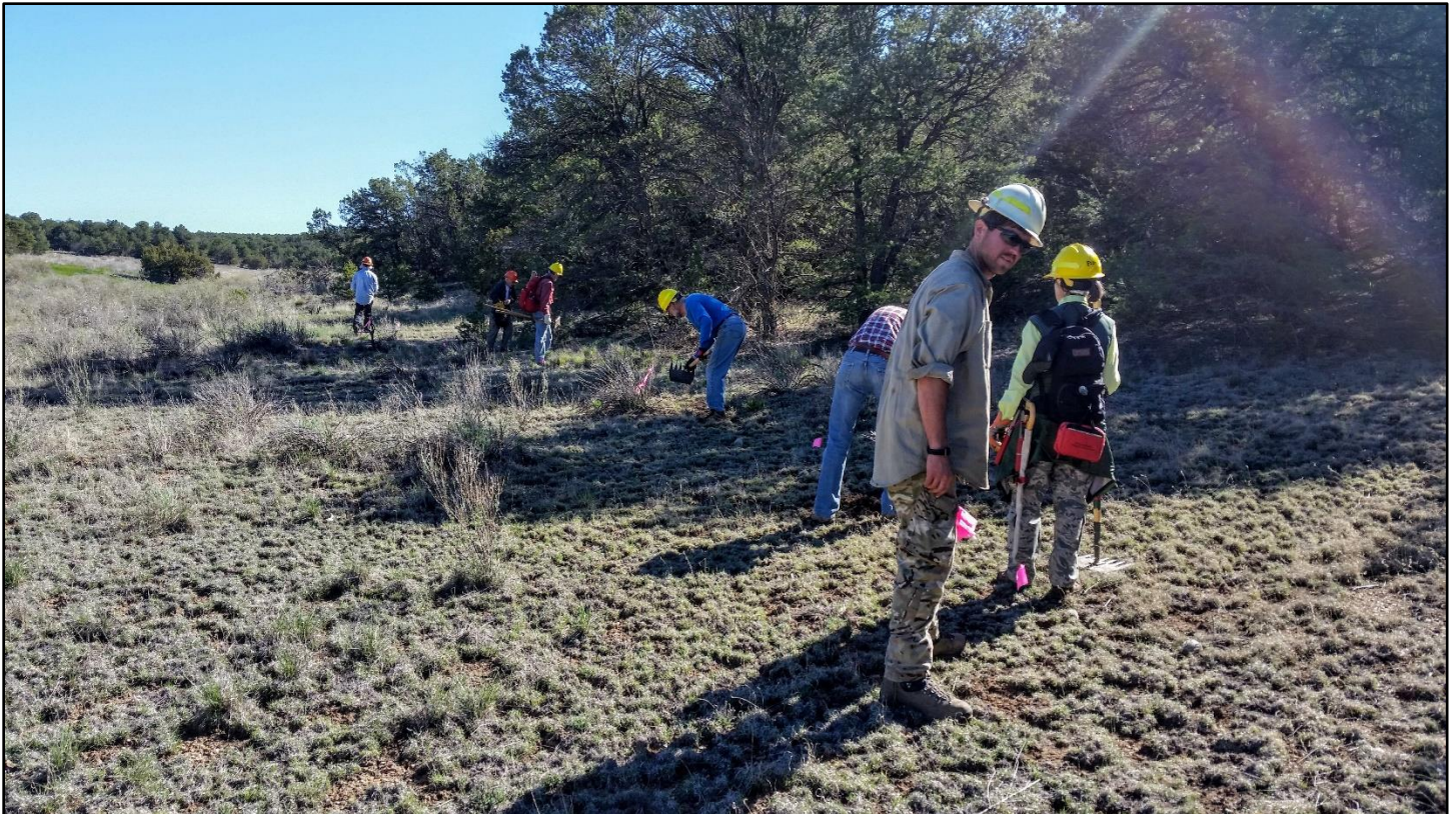
Up at Chamisoso, the boss eyes the flag line as the crew strings out to cut tread.
