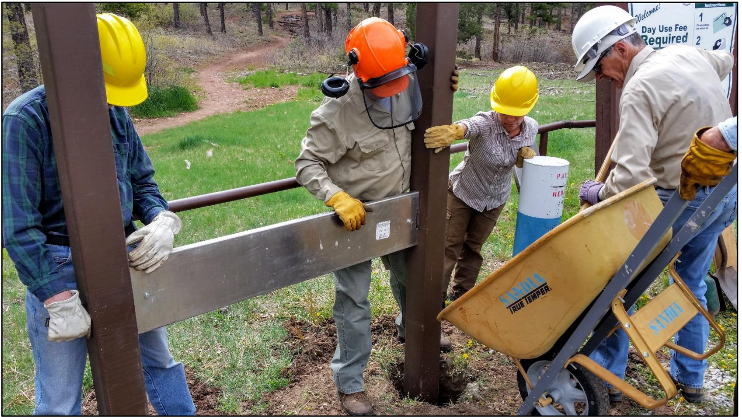
Mud in the hole. Keep those posts plumb!
