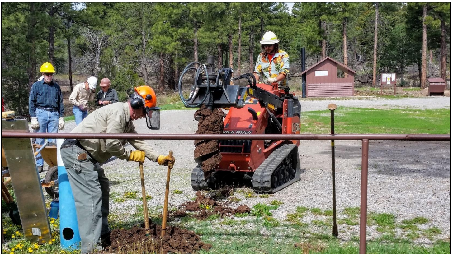
First hole: Surprisingly, no rocks to fight but damp dirt got packed hard on the auger.
