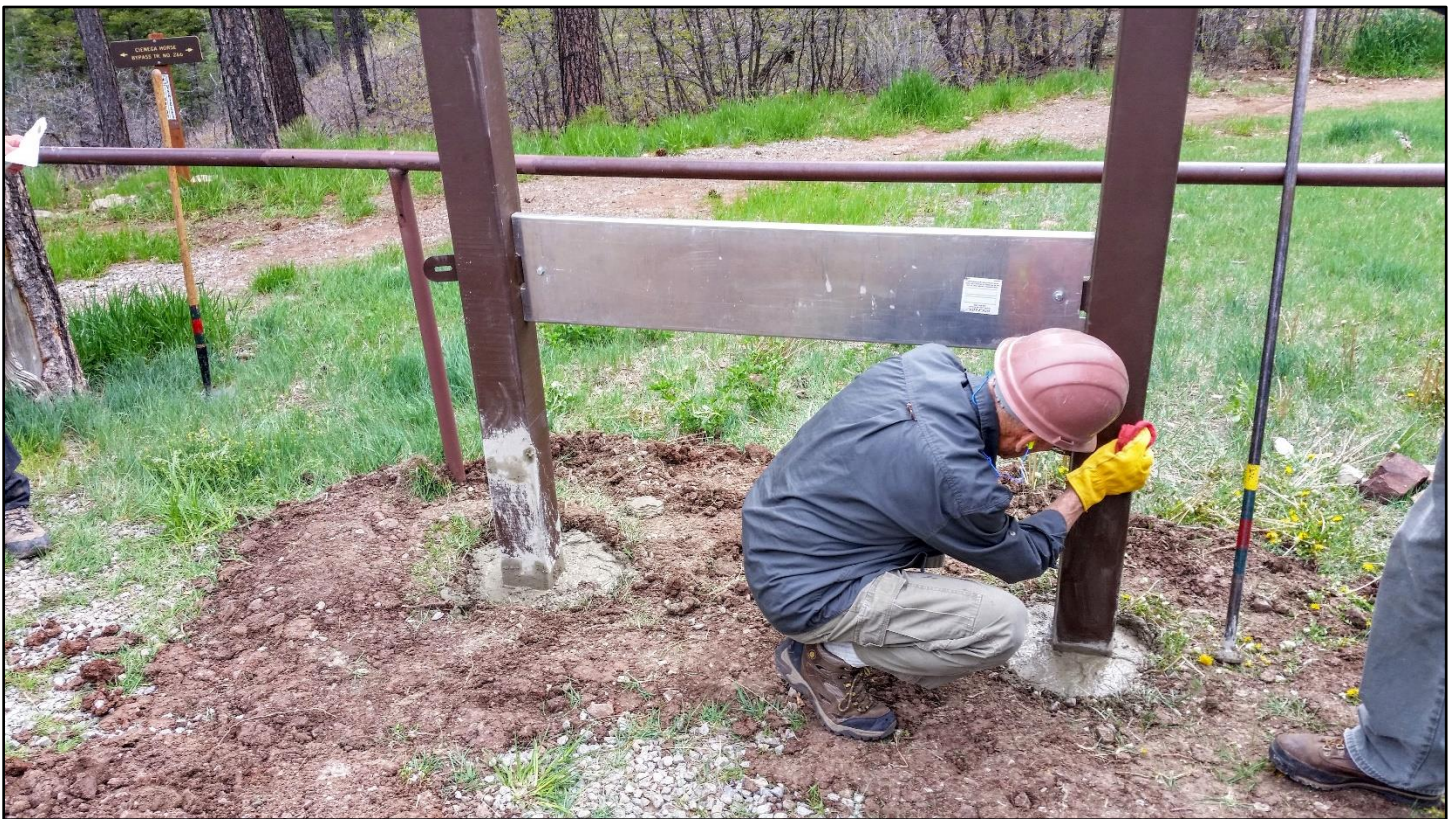
Let's clean off the sloped concrete. These posts are expensive.
