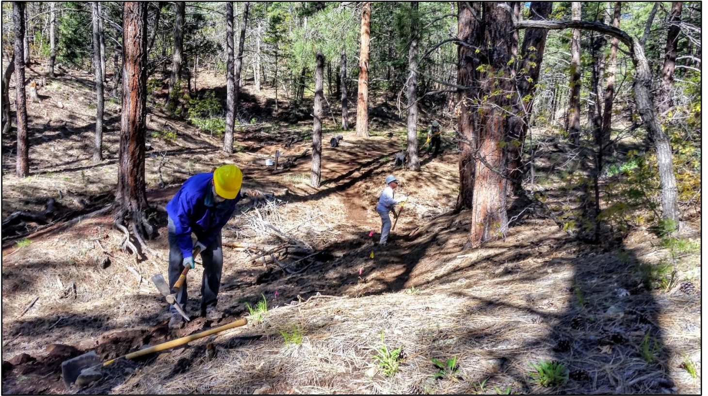
Meanwhile, the rest of the crew cuts in the upper end.
