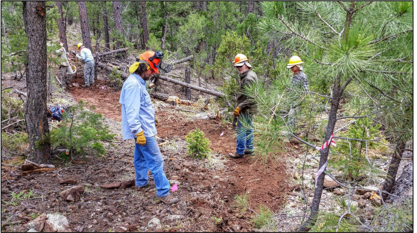
Turns in the trail are just hard to cut in. Not too steep, keep a nice line, ensure drainage.
