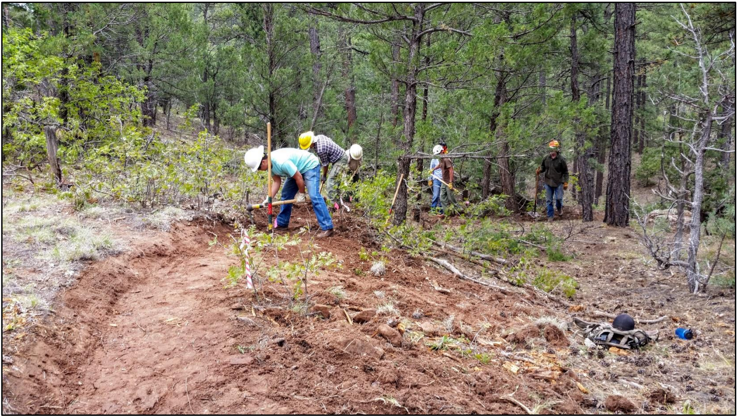
With the final line selected, the crew cuts in the turn and finishes the section.
