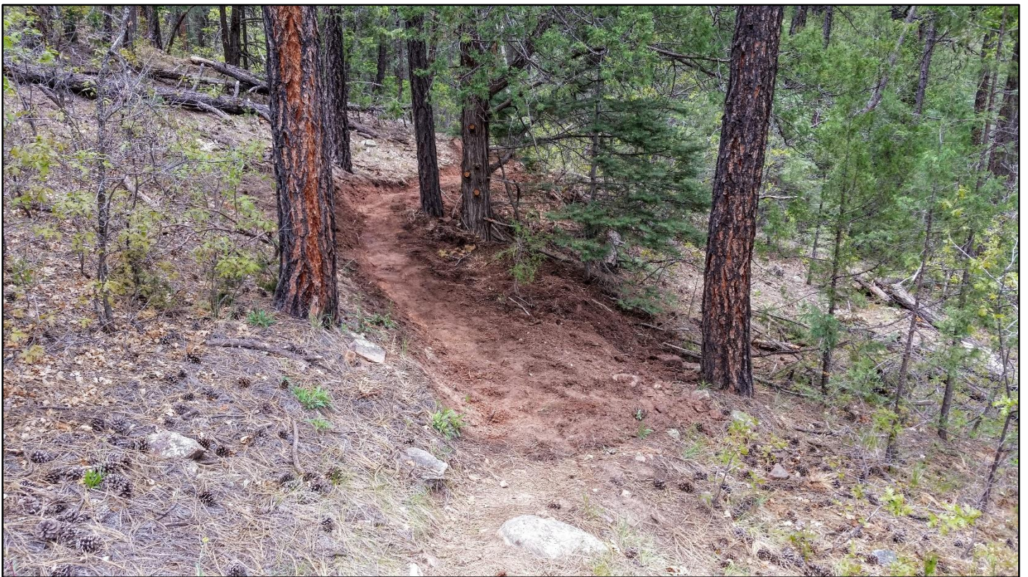
The upper connection of the loop is cut back into the user trail and the fall line section is obliterated.
