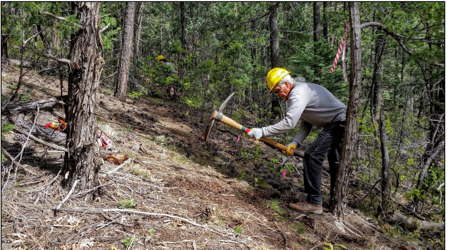
Get er' done! Starting to cut in the new line.
