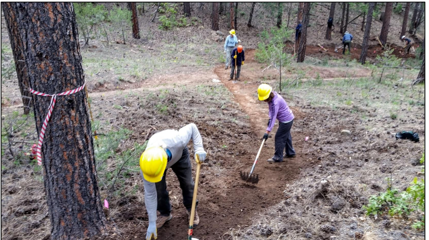
The new trail section is cut in and finishing touches are applied.
