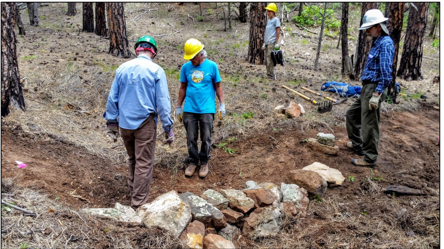
The rock crew analyzes the last drainage crossing of the day.
