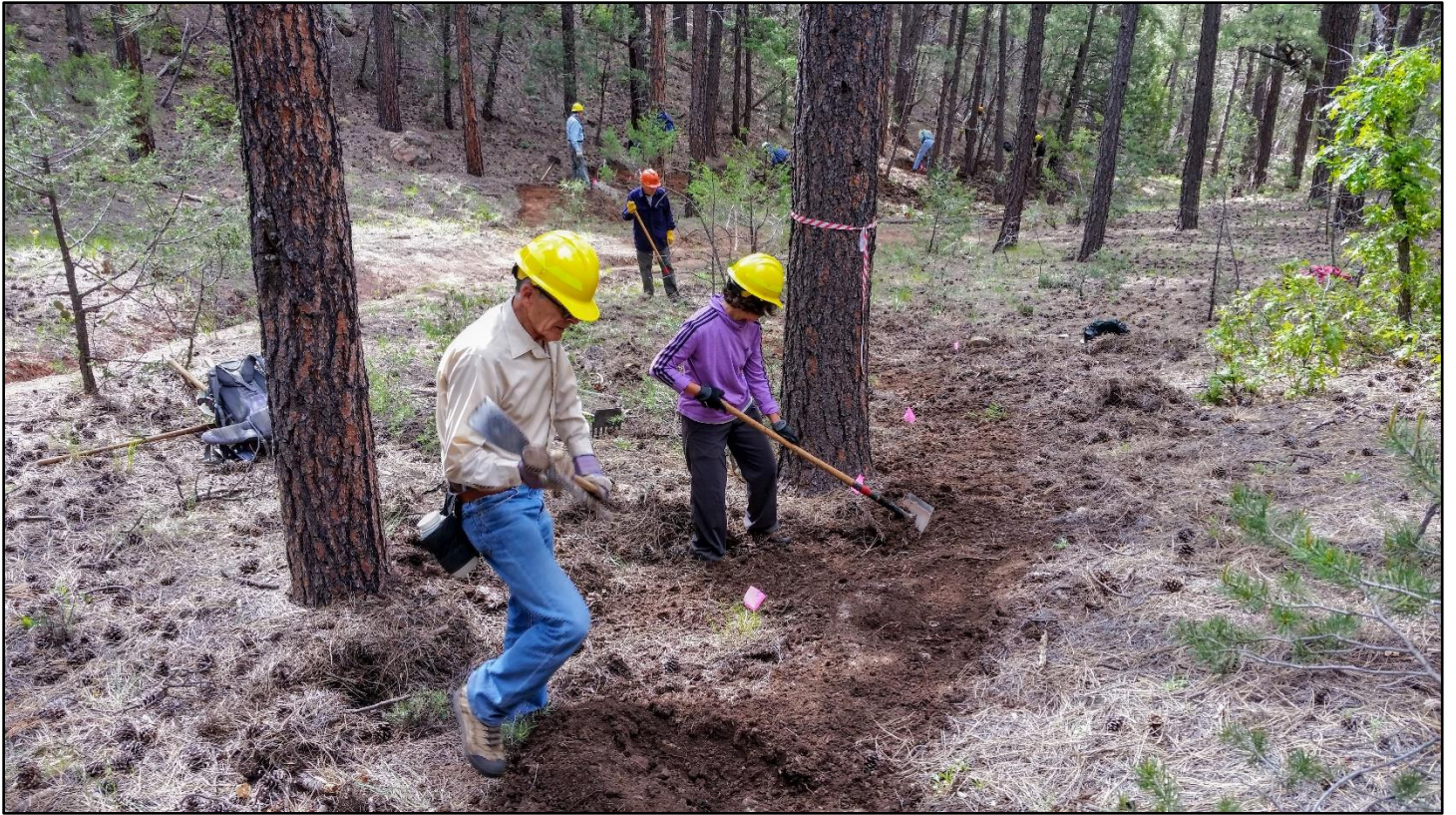
The thick duff is cleared and the new tread starts to appear.
