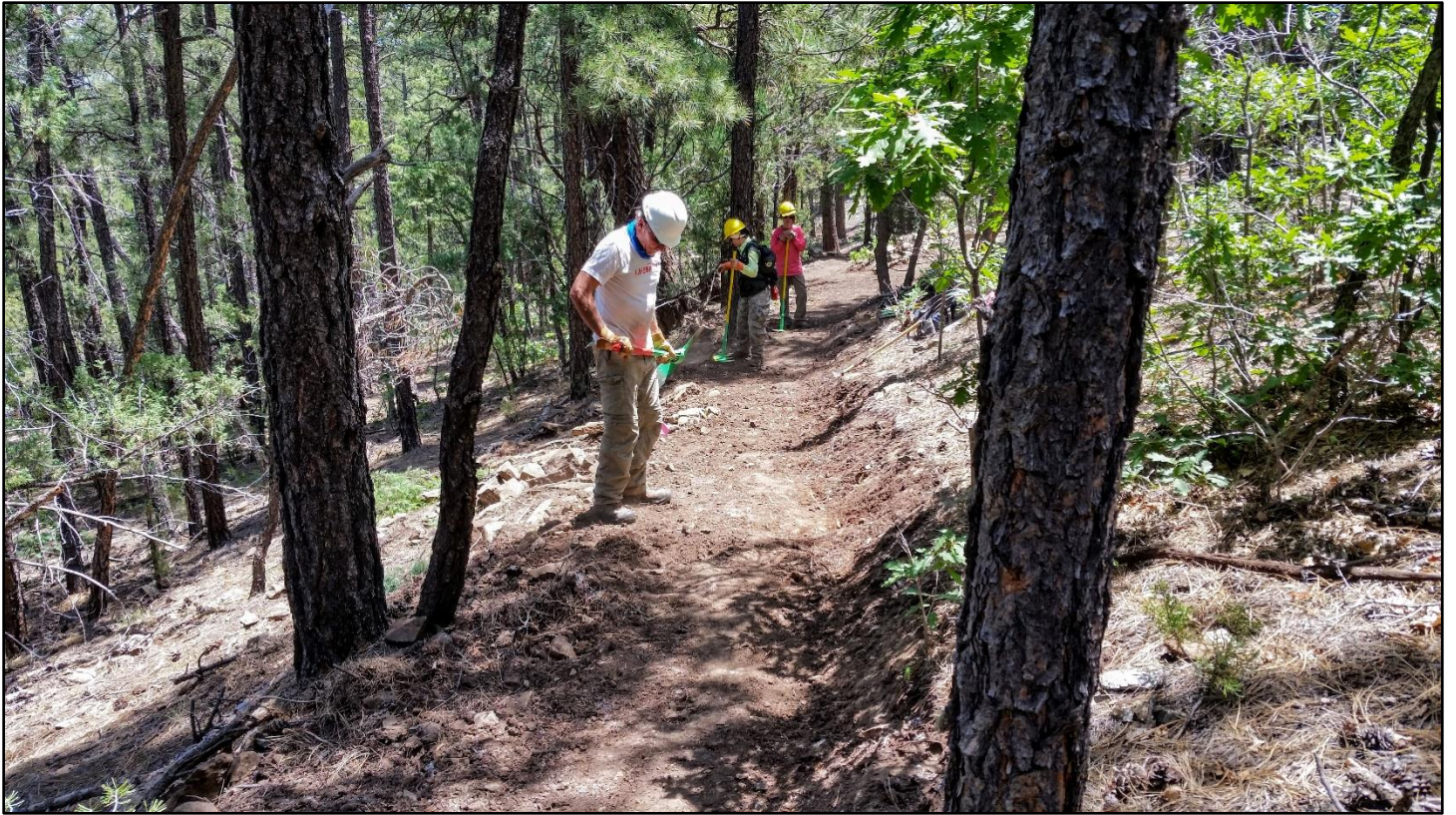
Behind the rough-in crew, the finishers create nice tread.
