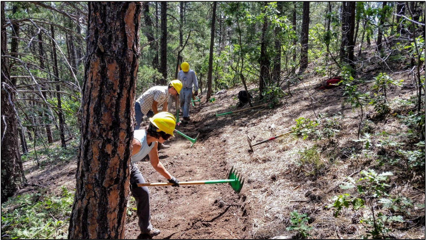
The crew starts to work their way up TC06.
