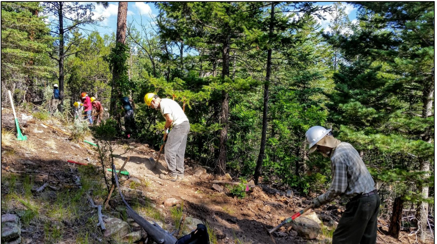
The crew lined up to level the new tread.
