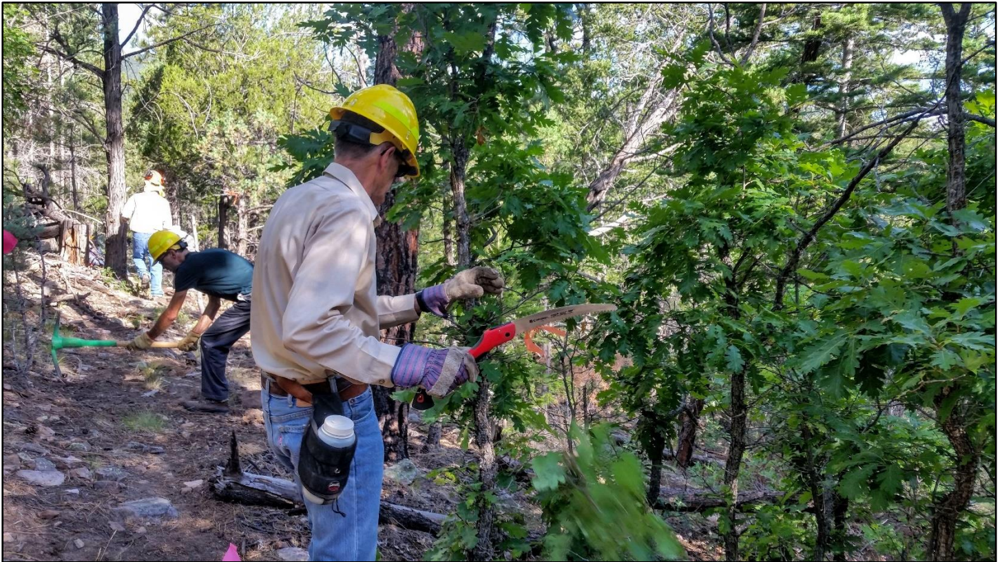
A little corridor clearing was necessary all along the line.
